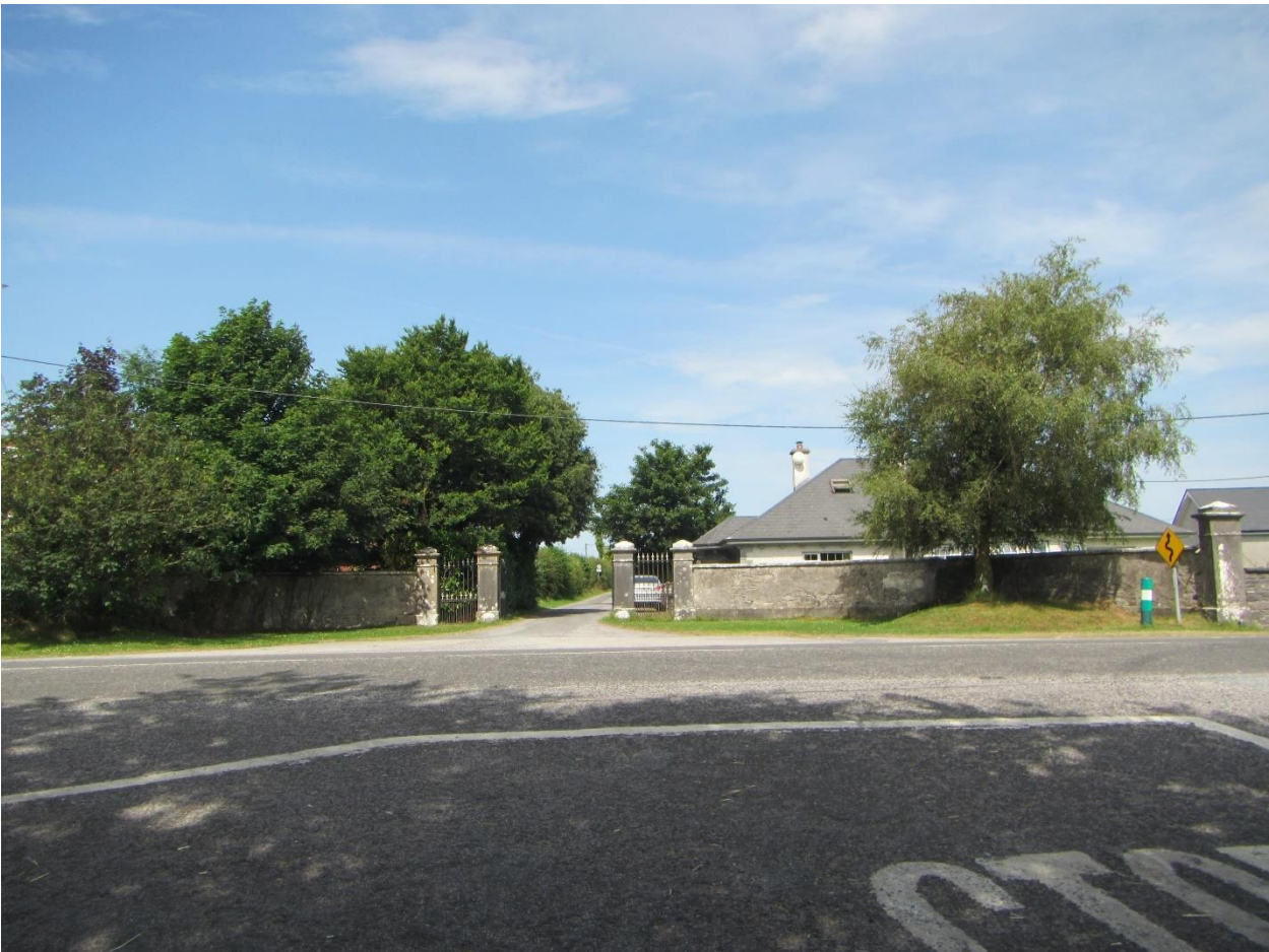
Photograph 8.11 The entrance gates to Rathmore House (RPS 3657) located on the north side of the N65.
