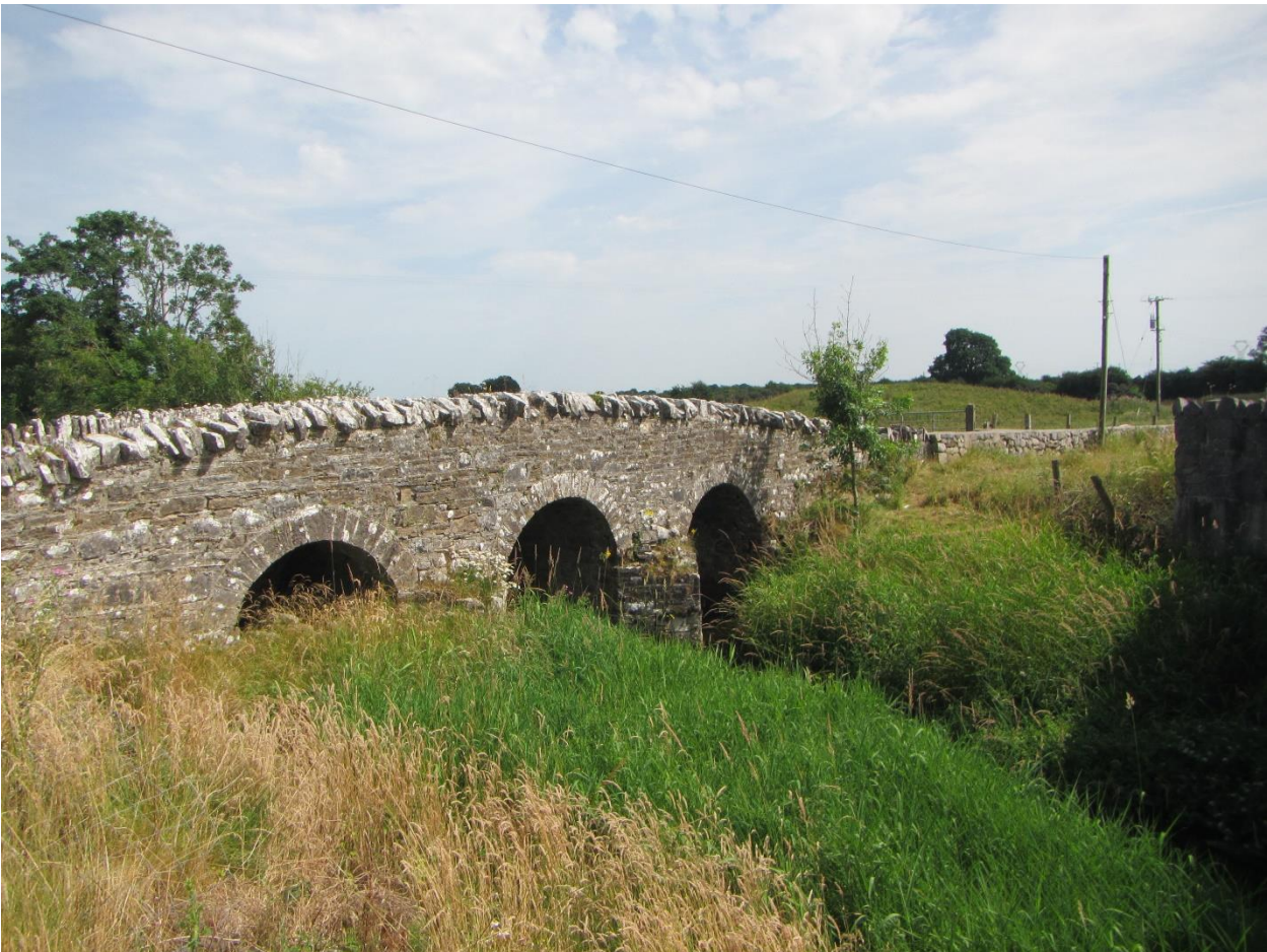
Photograph 8.9 Castletown Bridge (RPS 3651).
