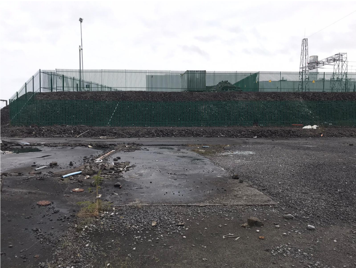
Photograph 8.2 Example of hardstanding within the Site.
